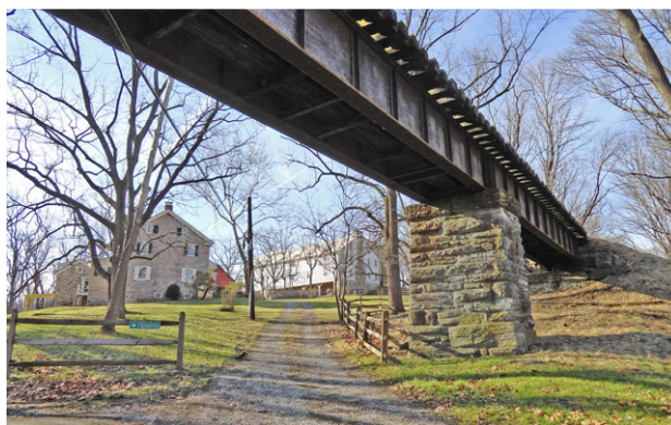
Bridge over Buckwalter Farm Lane in countryside of Charlestown Township
