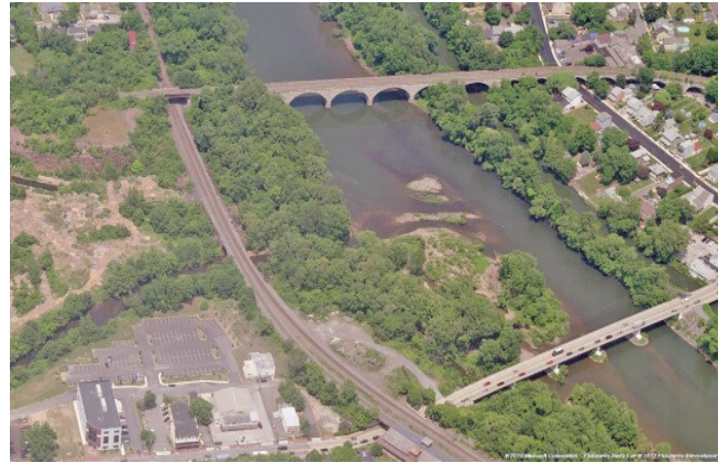
Norfolk Southern Railroad Bridge over Schuylkill River (top); Bridge Street / State Route 29 bridge (bottom)
