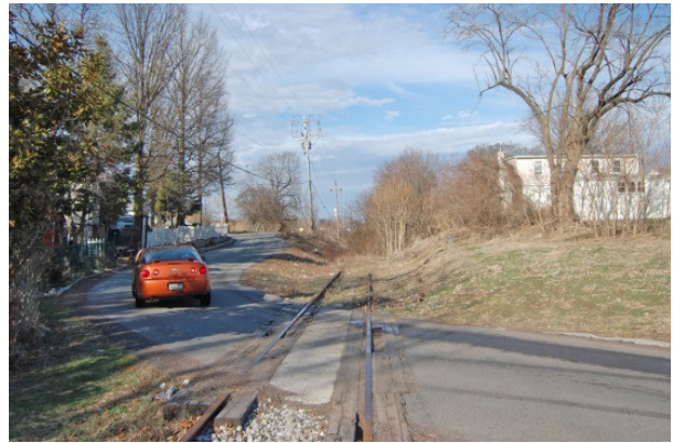
Railroad grade crossing of Montgomery Avenue
