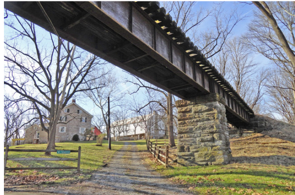
Railroad Bridge over Buckwalter Farm Lane
